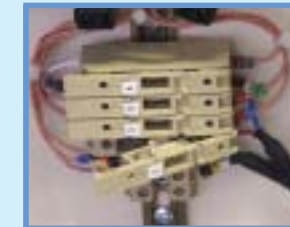
Detail showing both fuse box covers removed enabling easy access to the fuses
